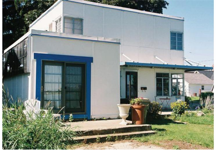
Motohomes were cutting edge prefabricated residences. They were composed of fiberboard panels measuring four feet by eight feet and then covered in an asbestos and concrete mixture. Some sources say cork, not fiberboard, formed the core of the asbestos and concrete mixture. These panels were connected by steel studs. (continued on page 4)
